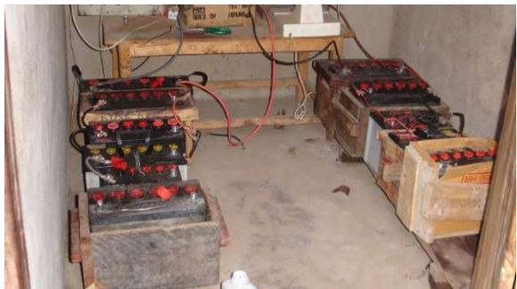
Fig. 17. Perhaps most innovative of all, investing in a generator to charge old car & truck batteries for neighbors to use in lighting home, listen to music or even watching videos on TV.
