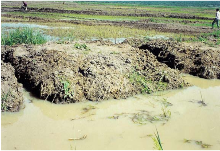
Photo 8.8 Gullies allowed to be eroded into a main drain in the Madibira project in Tanzania.
