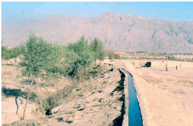
Photo 8.2 Lined irrigation canal in Pakistan as part of an On-Farm Water Management Project. Photo Credit: W. Shaner.
