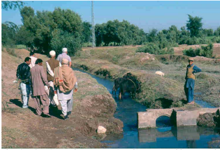
Photo 8.7 Once-improved watercourses in Pakistan managed by a WUA, but with the concrete turn-out, installed by the On-Farm Water Management Project that mandated the WUA, eroded out and functionless. Photo Credit: W. Shaner.
