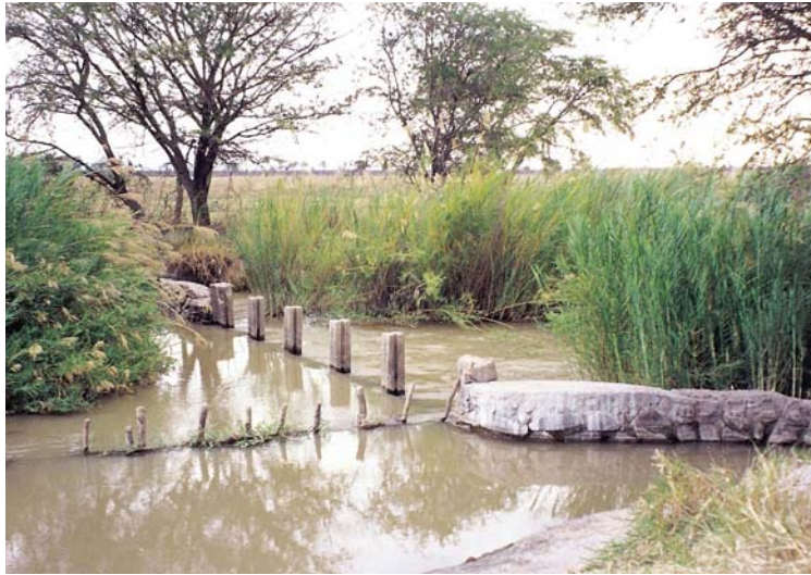
Photo 8.3 Concrete diversion into informal irrigation scheme near Madibira in Tanzania.
