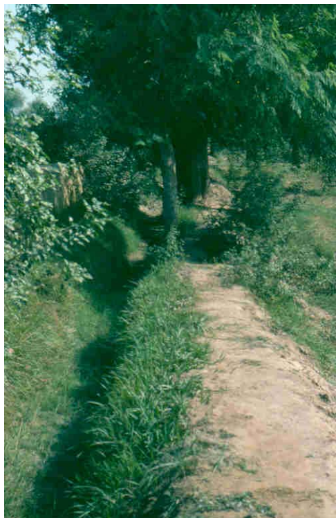
Photo8.6 Typical weed-filled watercourse in smallholder irrigation scheme. This photo is from Pakistan. Photo Credit: W. Shaner.
